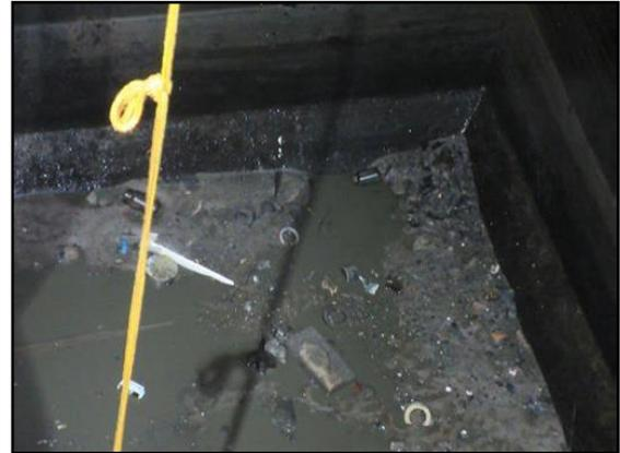
***Residual sludge and miscellaneous debris in Sludge Retention Tank 3 in WILWREP***
