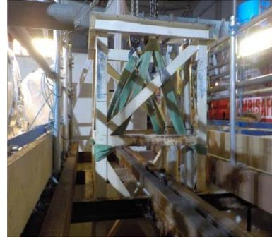
Lattice frame raised using the porta-gantry
