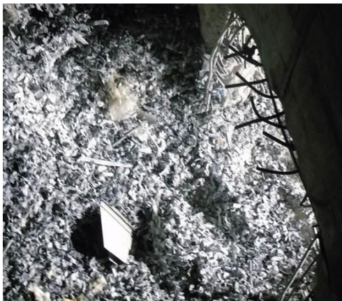
A view down into Bunker 1 showing waste just inside the penetration from Bunker 2
