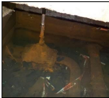
Rainwater filled chamber
