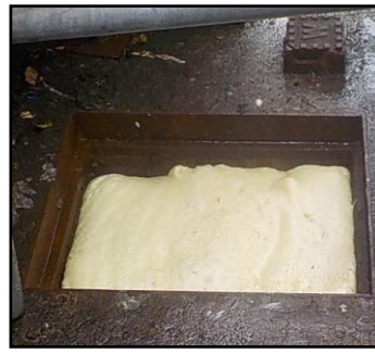
Foam filling of chamber
