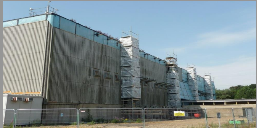
Building now ready for demolition
