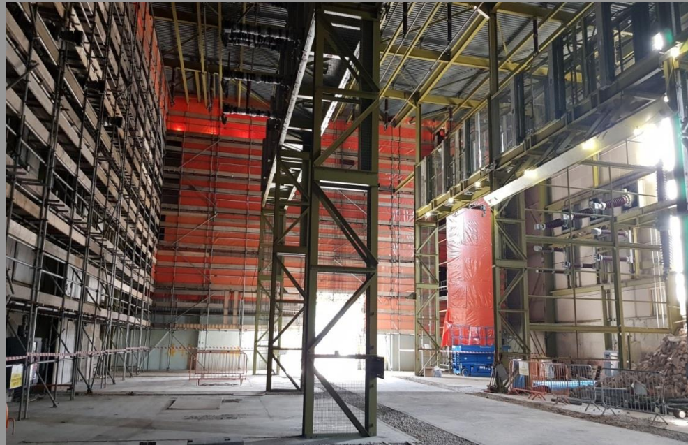
Scaffold to the east end of building
