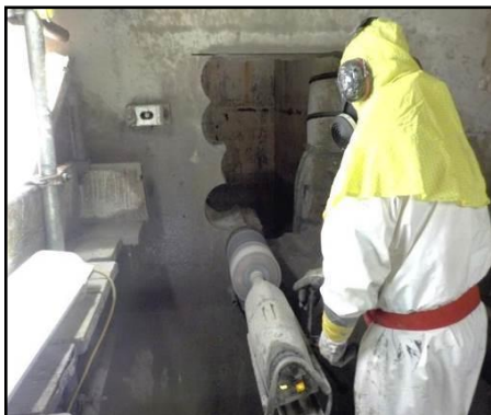
Coring rig in operation at a tank opening View of access doorways between the tanks
