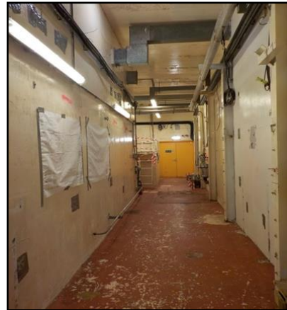
PWTP valve gallery with all redundant pipework systems deplanted
