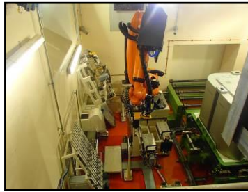
Grout plant modification phase
