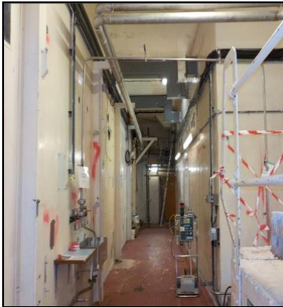
PWTP valve gallery with all redundant pipework systems deplanted
