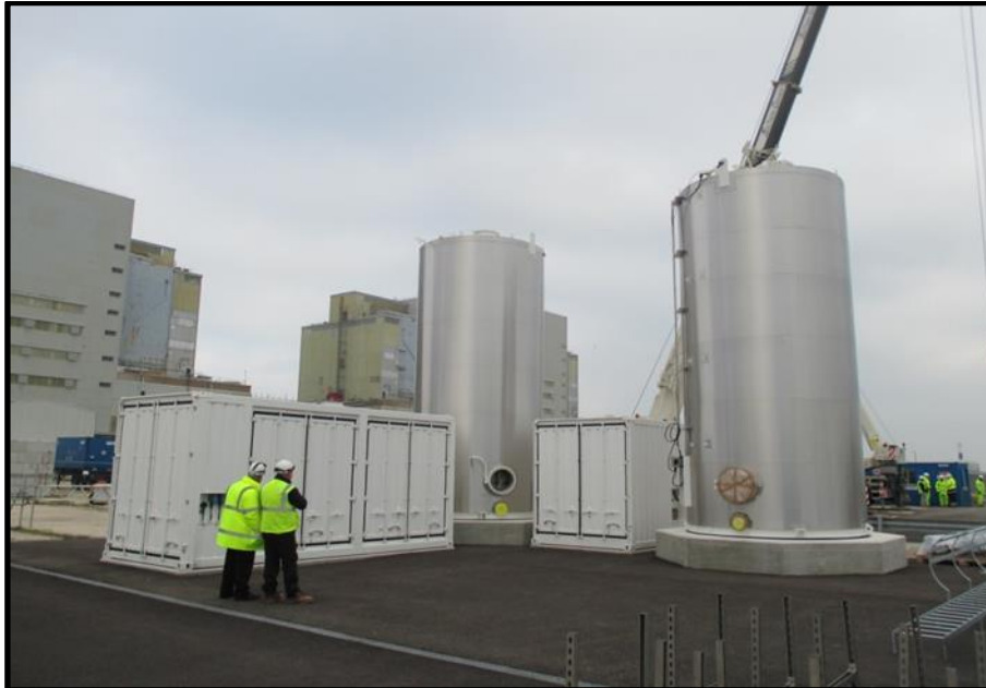
Installation of the MAETP
