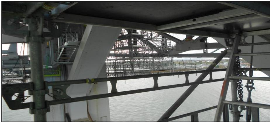
*This photograph illustrates a temporary works suspended access platform underneath the road bearing surface of the Forth Road Bridge at a height of circa 70m. During the visit C Spencer demonstrated fit for purpose management systems for controlling access to the temporary works.*
