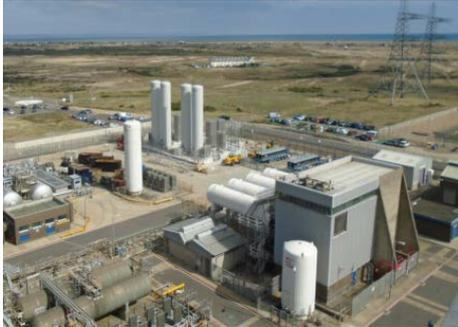
We are also in the process of building a **new nitrogen storage and injection system** (left). The station would use nitrogen as part of its safety systems. The existing nitrogen system has been in operation since Dungeness B was first commissioned and due, in part, to the recent extension of operating life of the station, needs a modern equivalent which will be in place in early 2019.
