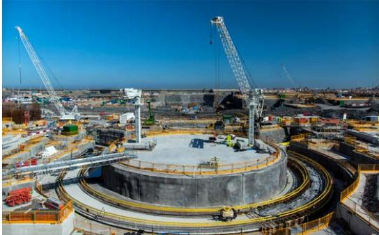
Work is advancing on reactor one with completion of its pre-stressing gallery: this structure sits below the reactor unit and will help to strengthen the main reactor building. The 'Deep dig' is now complete for Unit 1: this vast excavation is 21m below sea level and will contain the 54m tall water pumping station.
