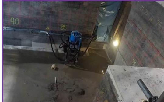
Ultra High Pressure (UHP) water jetting in the West Blockhouse tunnel has been completed.
