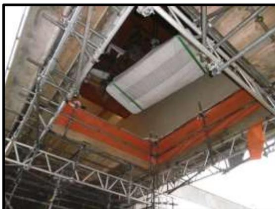
Removal of a 3 tonne (1 of 3) LLW steel gate from reactor two pond building
