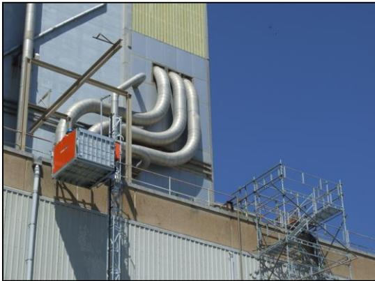
Mast climber and scaffolding erected to give access for boiler asbestos stripping
