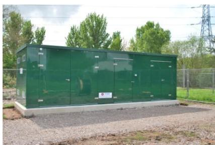
The new electrical sub-station just inside the site gate has been constructed and energised, currently feeding the Oldbury Technical Centre through the 11kV line from Alveston.
