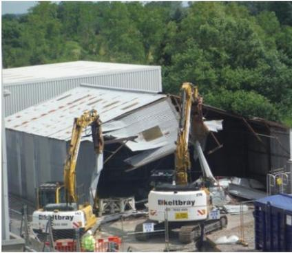
The redundant mobile crane store on site has been demolished. Contractors Keltbray removed internal tin sheets and insulation before the structure was taken down using two 360 degree excavators with grab and pincer attachments. A total of 39 tonnes of metal was sent for recycling.
