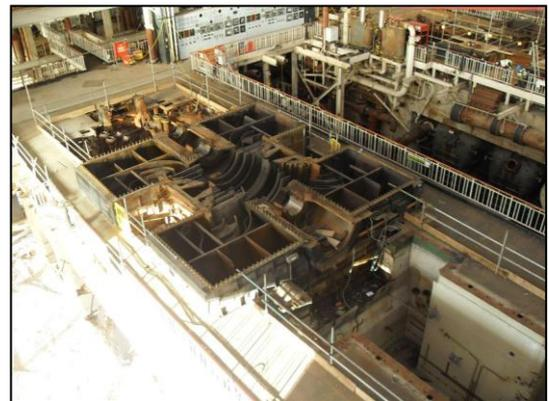
A turbo generator stripped down to the steam chest
