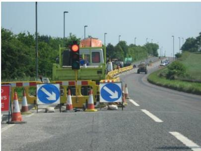
Those local to Thornbury will have noticed roadworks working their way northwards from the electrical sub-station at Alveston. This is the start of the journey for an 11kV cable that will eventually end up at site, allowing the 132kV lines from Iron Acton to the site to be made redundant.
