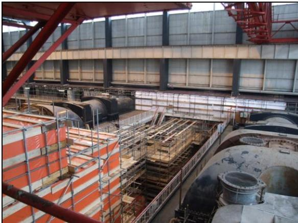
Asbestos enclosures under construction in the Turbine Hall
