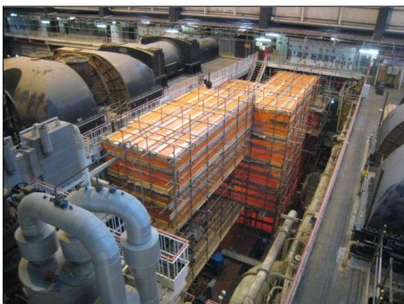
Asbestos enclosures nearing completion
