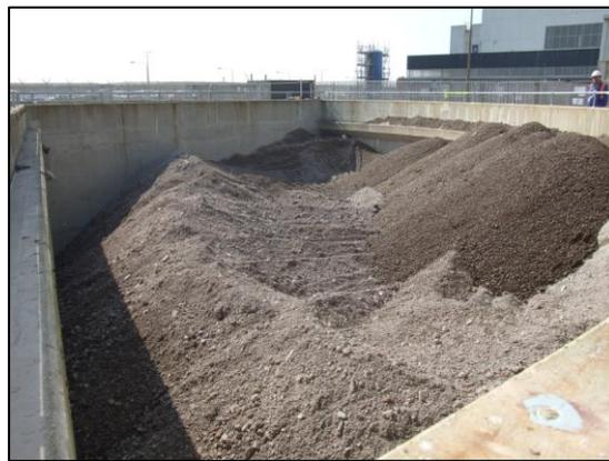
Concrete rubble and shingle from site used as infill for the CW pumphouse
